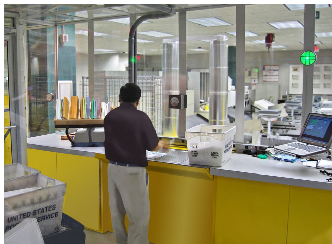
An operator sorting mail over a downdraft table. ASAP III control software runs on the laptop, while detection instruments are installed under the counter.
