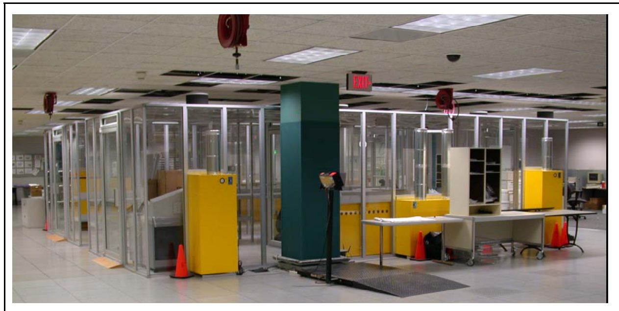
Installed Negative Pressure Mail Room (NPMR).
