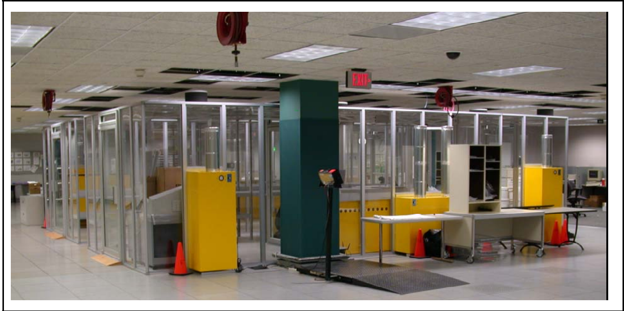
Installed Negative Pressure Mailroom (NPMR).
